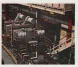
Air cooled steel cylinder mercury are rectifiers were first developed in 1946, and many have been supplied for railway traction service as instanced by the 2,500 kW 1,500-w/ot sub-station equipment pictured at left undergoing Works tests. Bull in 1952, it is one of several air-cooled equipments for British Railways.
