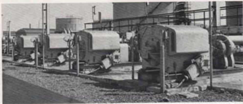
Surface-cooled flameproof induction motors driving high-speed pumps at an Australian oil refinery.
