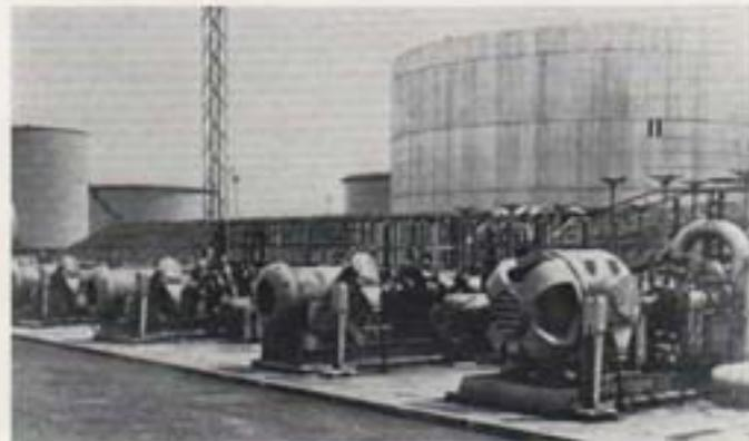
A large tube-cooled and smaller surface-cooled flameproof induction motors driving pumps at an oil refinery.
