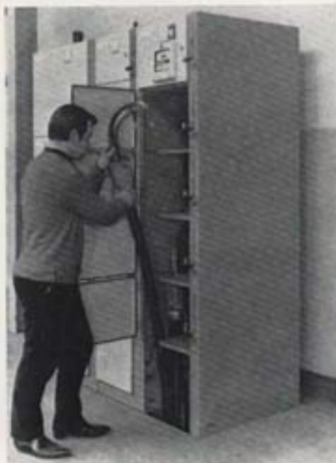
Top right, a type 'T' air-break circuit-breaker for systems of 3kV up to 17.5kV partially withdrawn from its housing. A switchboard of these circuit-breakers for a 6kV 300MVA system is also illustrated.
