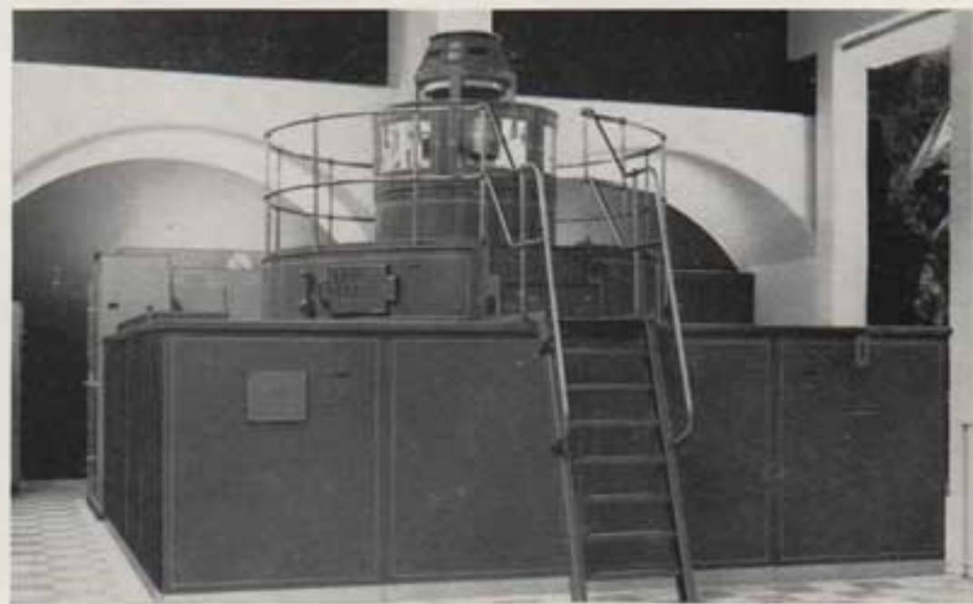
21 MW 600 r.p.m. 11 kV closed-air-circuit water-cooled synchronous generator
