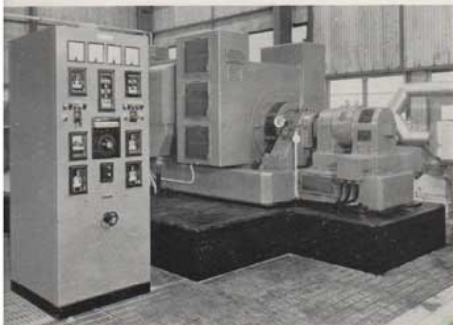
4000 h.p. 1500 r.p.m. 11 kV filter-ventilated salient-pole synchronous motor driving a centrifugal compressor at an oxygen plant
