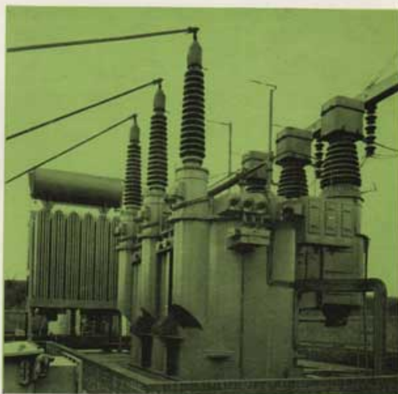
120/240 MVA 275/132 kV ON/OFB-cooled transmission auto-transformer
