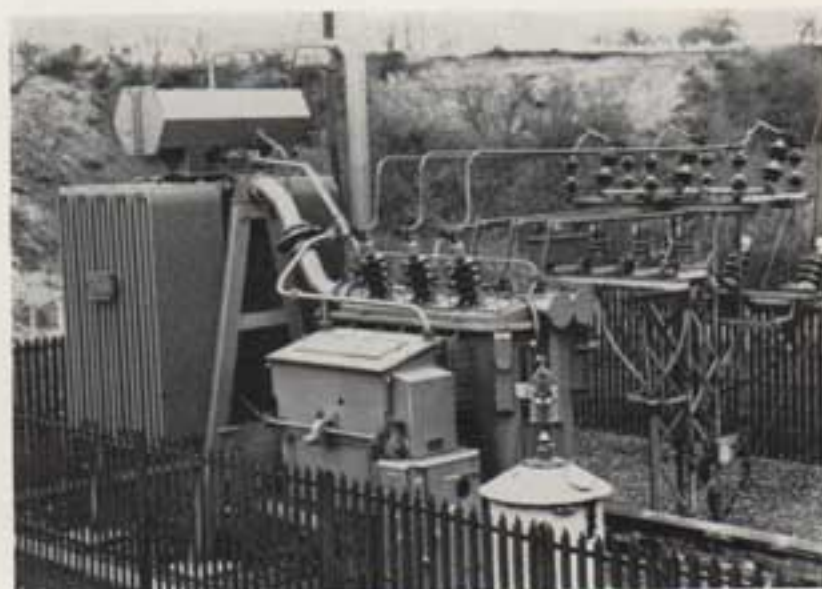
10 MVA 33/11 kV ON-cooled system transformer
