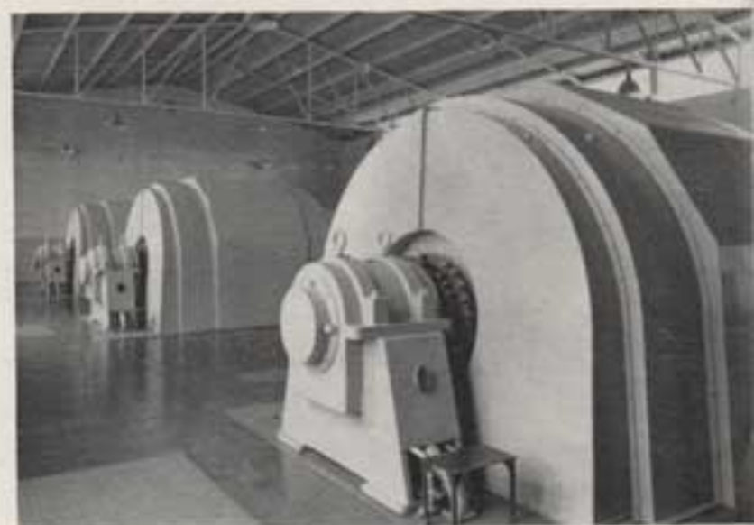
16.4 MVA 750 r.p.m. 12 kV closed-air-circuit water-cooled synchronous condensers
