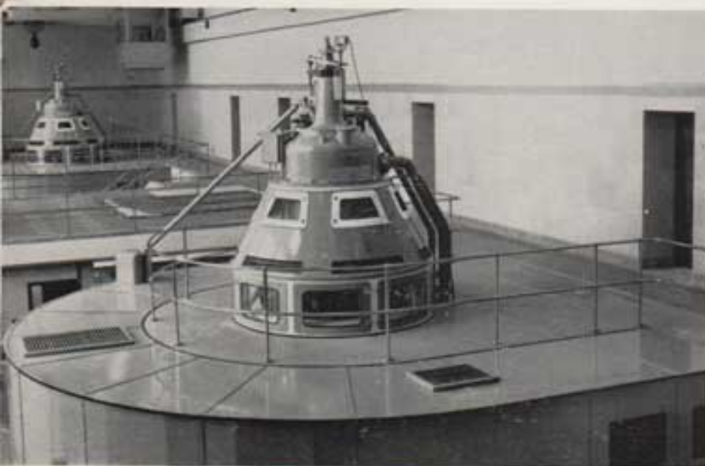
10 MW 187.5 r.p.m. 11 kV closed-air-circuit water-cooled synchronous generators
