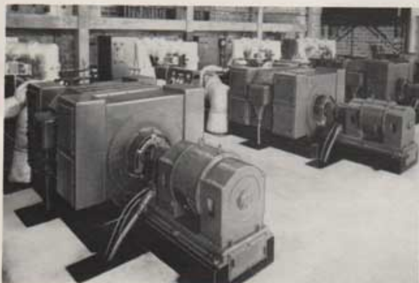
900 kW 1500 r.p.m. 2.4 kV geared gas turbine-driven filter-ventilated a.c. generators
