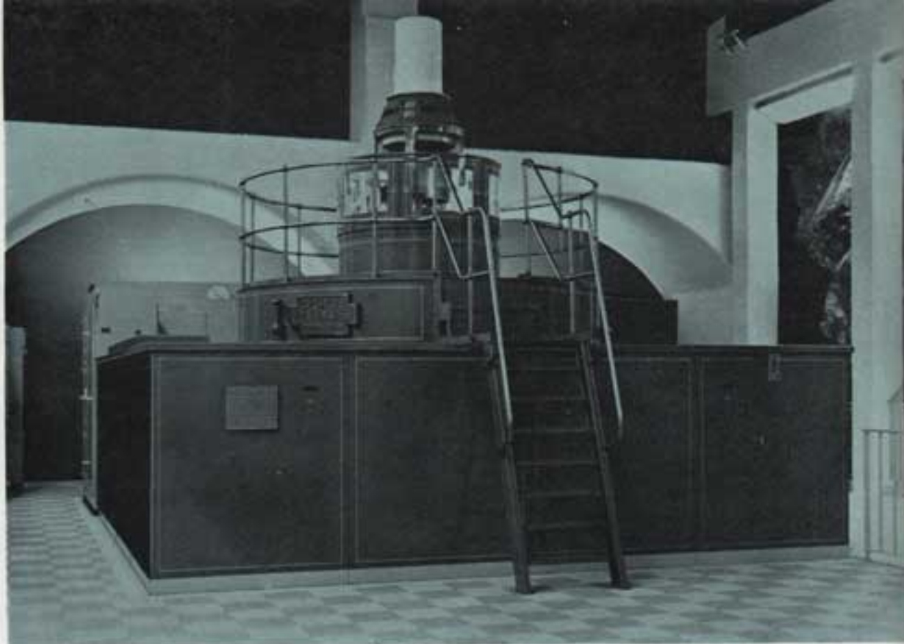
21 MW 11 kV 600 r.p.m. closed-air-circuit water- cooled vertical-shaft synchronous generator
