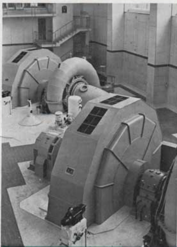
12MW 375 r.p.m. duct-ventilated horizontal-shaft hydro-generators
