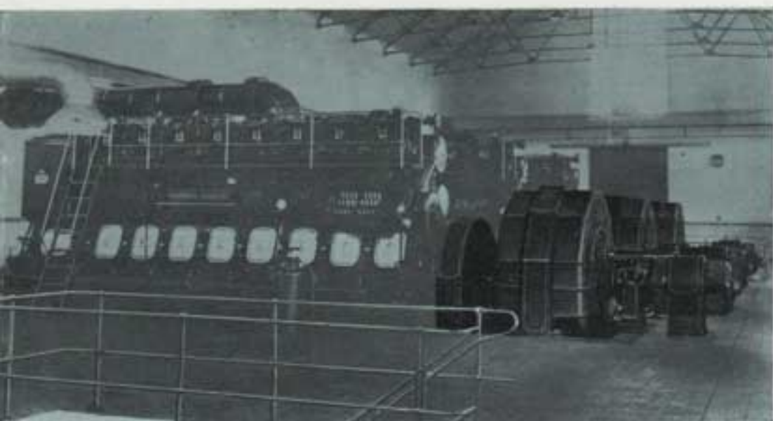
1000 kW 11 kV 300 r.p.m. screen-protected engine- driven a.c. generators
